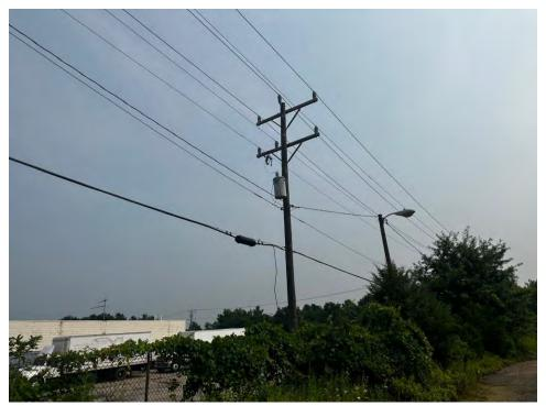
Photograph # 13 - Pole mounted transformer on eastern property line (7/13/2023)
