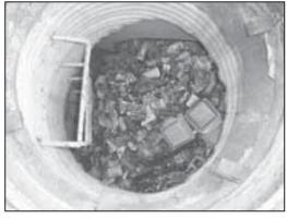
Trash and sediment can quickly accumulate in underground detention facilities, requiring frequent clean outs, by professionals.
