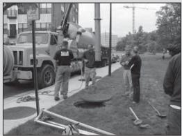
A vacuum truck may be required to remove sediment from stormwater facilities located underground.
